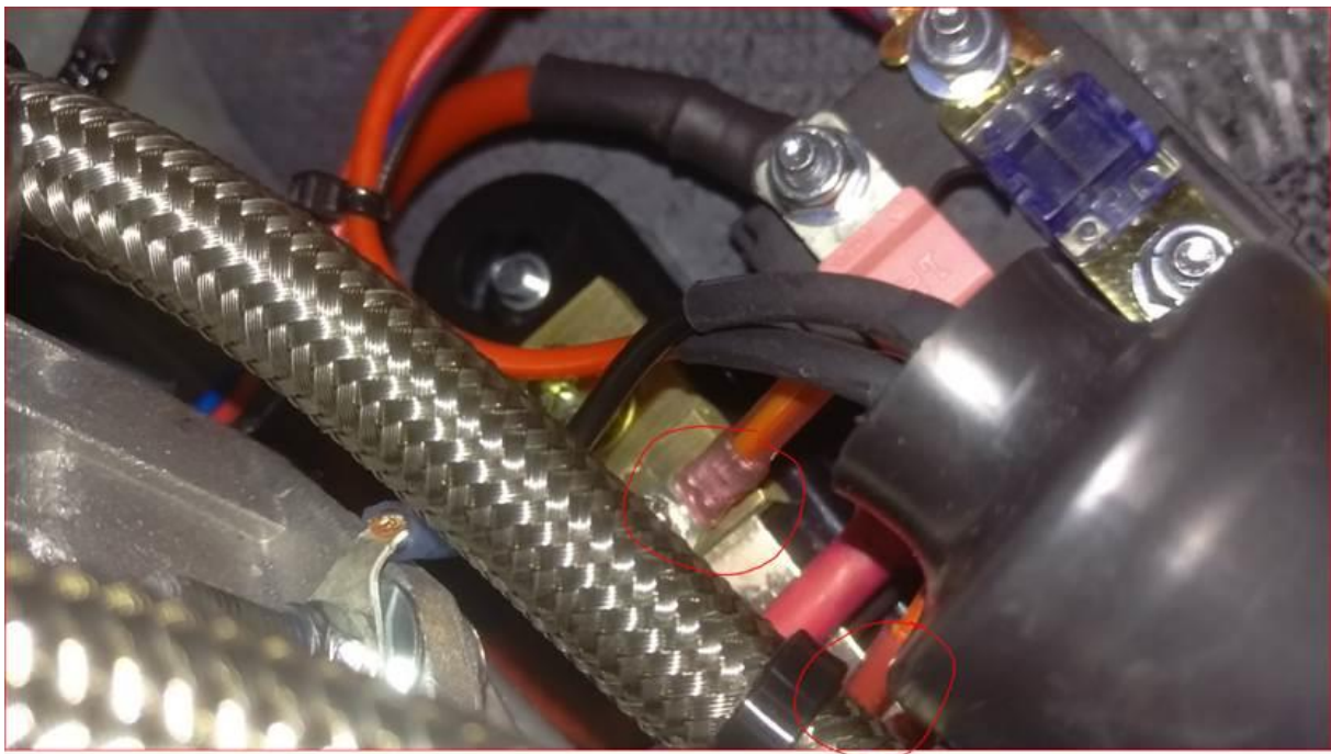
Fig 4: Shunt, new Installation
