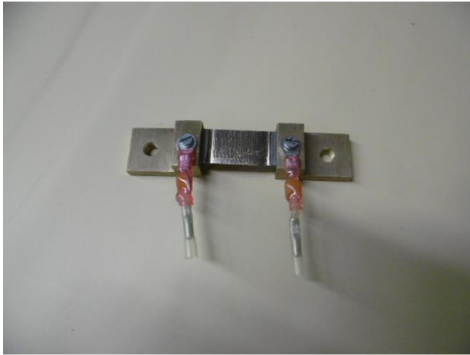
Fig 3: Shunt, new installation
