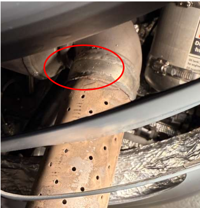
Cracked welding seam, after muffler lost
