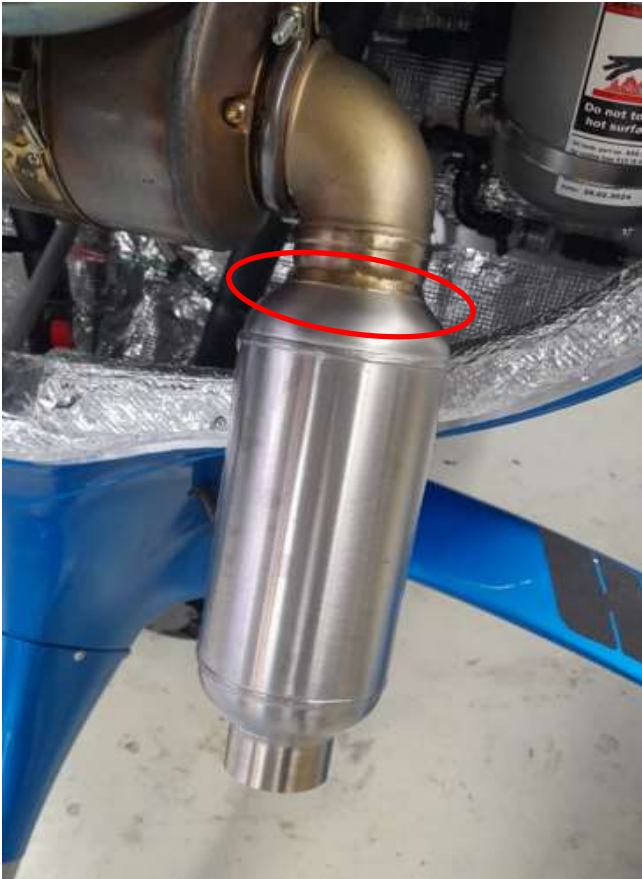
Welding seam which has to be checked
